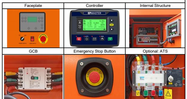
It has a digital LCD screen, which provides easy reading of the information regarding the Engine, Alternator, Mains and Charging. The controller meets all requirements for Auto Mains Failure (AMF) applications including remote communication and internet control, user configuration and complete genset monitoring and protection.
